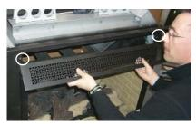
Attach the Bottom Louver or Grill to the hinges on the bottom flange of the fireplace.
