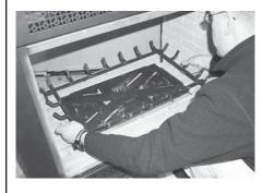
4) Remove the burner assembly by removing the 4 Phillips head screws and then slide the burner assembly away from the orifice and lift out.
