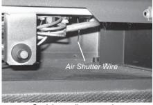
Straighten adjustment wire.
