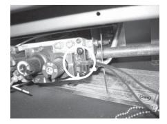
**31)** Locate the ground lug at the receptical box, left of the unit.
