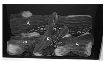
7) Place the center cross log on the locating pin in the top of the rear log and position as shown below.
