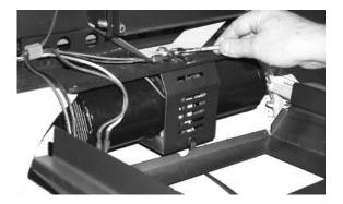
12) Before re-attaching the rear access panel, the valve wires and the fan wires need to be connected.
