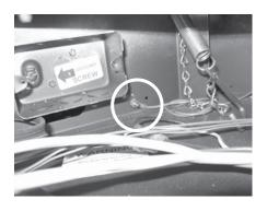
6) Connect one end of the supplied green ground wire to the lug with the nut and washer from the kit.
