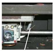
Adjustment Wire: Push to close or pull to open aeration cap.
