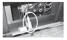
4) Plug up the Piezo Ignitor mounting hole with the plastic plug.
