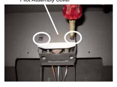
5) Remove the firebox base by lifting up from the back and maneuver out carefully. Ensure not to scratch the paint work or damage the pilot while lifting out.
