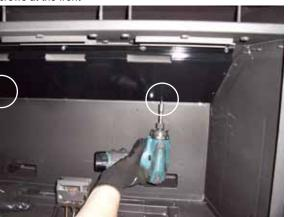
**10)** After the top panel has been secured - install the back panel. The back panel is held in place by the side panels
