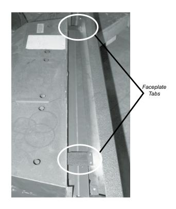
Secure the bottom of the faceplate to the firebox flange using one screw on each side.
