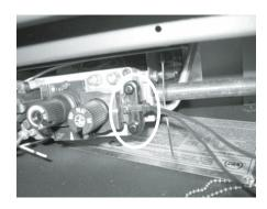
5) Locate the ground lug at the receptical box, left of the unit.
