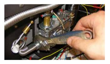
6) Disconnect the Gas Supply Line from the On/Off Safety Shut off Valve.
