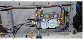
Loosen both screws at the top of the valve about ½ way out. Lift the valve body and lean outward. The Valve Brackets will rest open as shown on the right.
