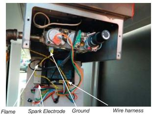
5) Remove 4 screws to remove DFC box.
