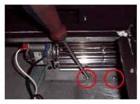
Attach the green ground wire to the ground lug – located in the lower left back corner of the unit.
