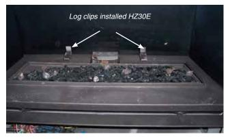
2. Position Back Log (1) by positioning centre of Log on centre of pilot hood.Rest Log 1 on log clips. Each end should rest on the lip of the burner tray – as shown below.
