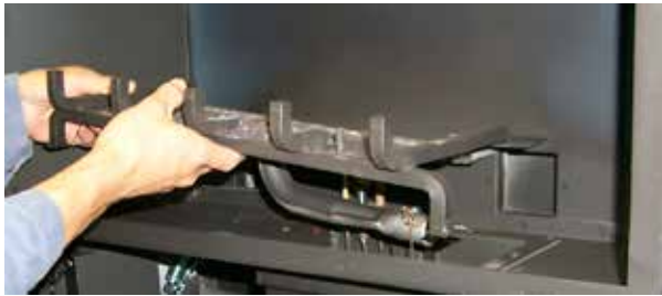
Diagram 1: Remove the left and right screws and then lift out the burner/grate assembly.
