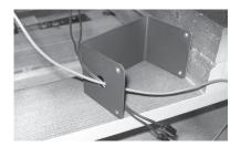
Install the plastic bushing over the outside of the hole.
