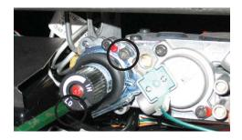
**10)** Install the stepper motor in the same location the hi/lo knob was removed from - with 2 screws as shown below.
