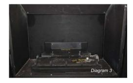
**3)** Install the top panel next - slide the panel in over top of the back panel - orient the panel so the fold in the metal faces in (see inset A).
