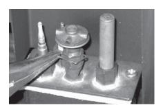
Pull off the pilot cap to expose the pilot 8) orifice.
