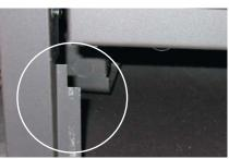
Diagram 3b Bracket on unit for bottom mesh door.
