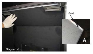
**4)** Remove 1 screw (see inset A), position right side panel in firebox - position panel clip in place and secure with 1 screw (see inset B). Tighten the screw.
