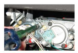
9) Install the ground wire to the ground lug just behind and to the left of the valve on the HZ42E and to the right of the valve on the HZ42STE.
