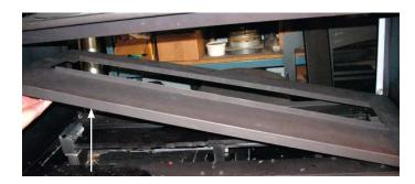
6) Remove burner by removing 2 screws.
