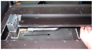
Remove cover plate located in the centre of the firebox floor by removing 4 screws. Discard the cover plate and gasket - keep the screws
