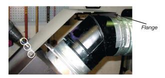
4) Install the extender on top of the deflector with 2 screws - slide the extender until it touches the outside wall - tighten screws to secure. Extender can be adjusted to max. 15-1/2".
