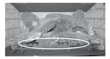
12) Place rock wool along side the embers on the front of the burner as shown. Ensure not to cover any burner ports.
