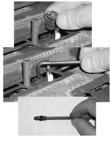
Remove burner orifice with 1/2" wrench.
