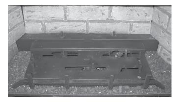
3) Fit log 27-23 into the pins on the back log tray.
