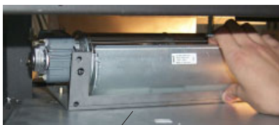
Position Fan B on mounting studs.
